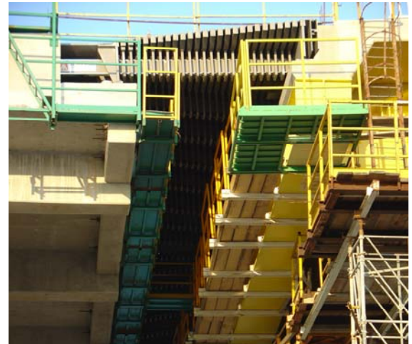
Fig. 1, 2: Installation of the Rion-Antirion expansion joint
